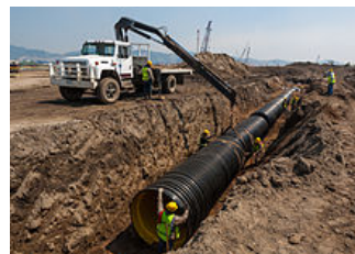
Figure 2: underground installation of agricultural HDPE pipe[6]
